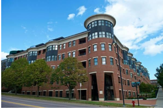
Central location at the corner of College St and Battery St
